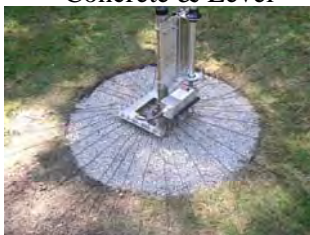
Radial Wires Installed Antenna Installed
