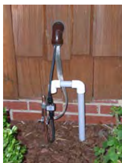
Shack end - Ground Rod and PolyPhaser protection
