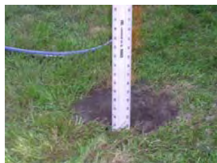
Hole for Mounting Pipe
